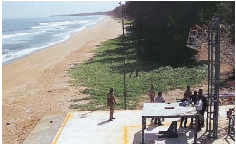
The facility has two sections, the launch pad and the Agnikul Mission Control Centre
